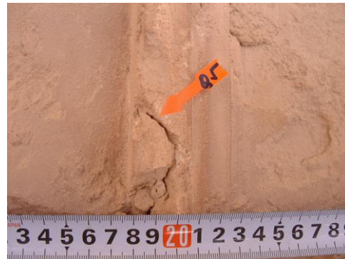
Stucco, exterior east facade
