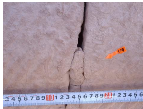
Joint mortar, exterior east facade
