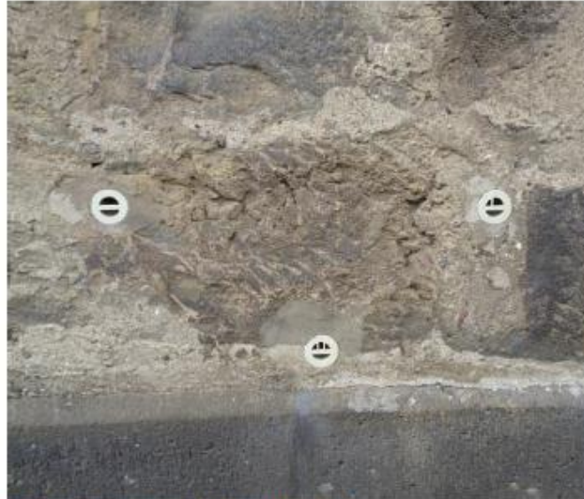
Figure 2, Different types of Knapen Siphons in a wall (Lubelli, B.)
