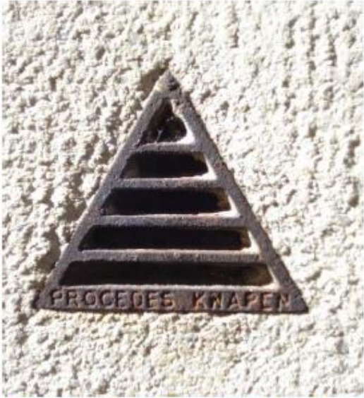
Figure 2, Different types of Knapen Siphons in a wall (Lubelli, B.)
