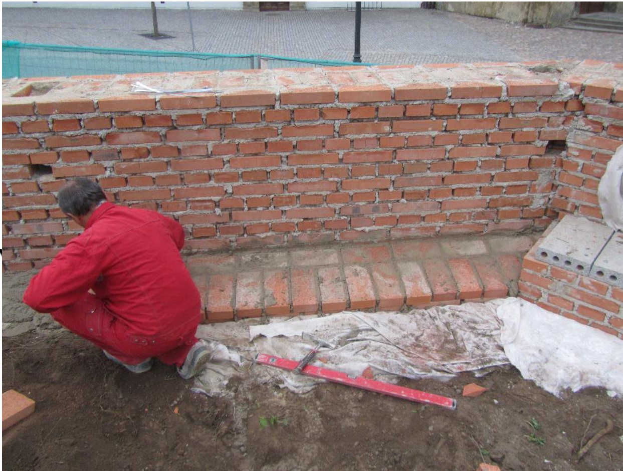
Wall reconstruction / rebuilding 2019/2020
